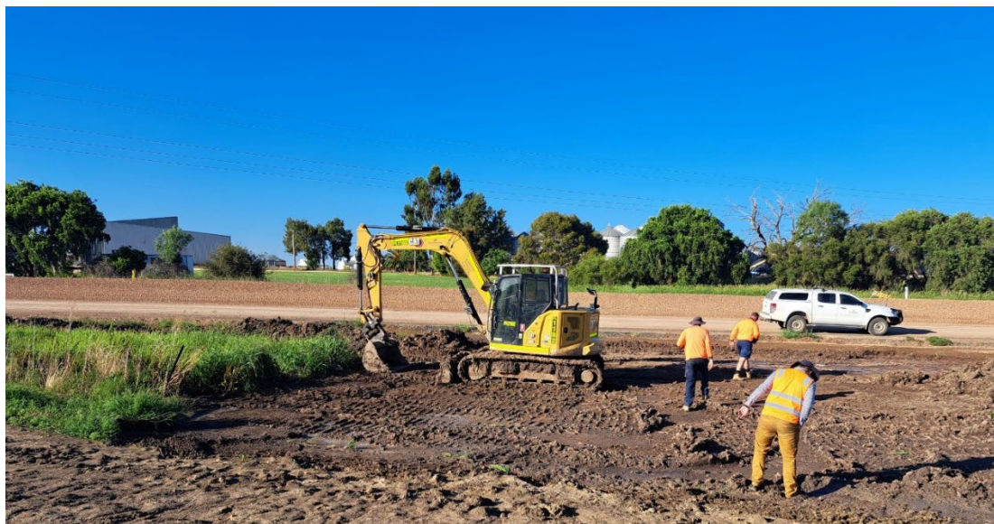
Figure 3: Works on Gainsborough Road are well underway
